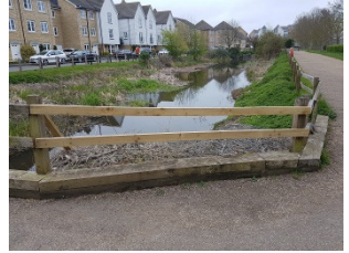
Fences Repaired Quickly
